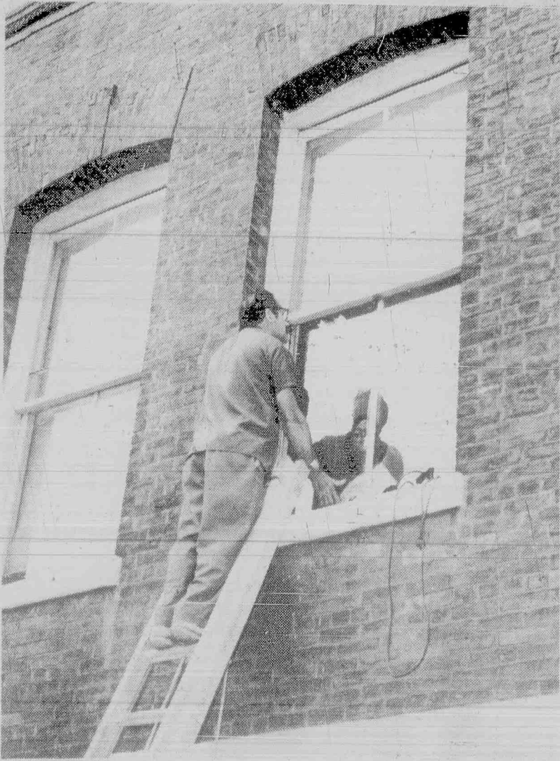
ONEUPMANSHIP — Board of Education carpenter John Przhocki and helper Jeffrey Goodfriend install specially constructed windows at School Three. The windows, made of clear plastic, will hopefully thwart vandals.
